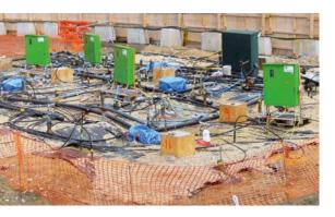
A total of **18,000 tonnes** of highly contaminated soil and groundwater have been successfully treated using a combination of ex-situ and in-situ remediation techniques, including **in-situ thermal treatment (ISTT)**. Here, we combined **SEE (steam enhanced extraction with air-co-injection; TUBA® method)** and **TCH (thermal conductive heating, THERIS® method)** for a highly efficient source zone
